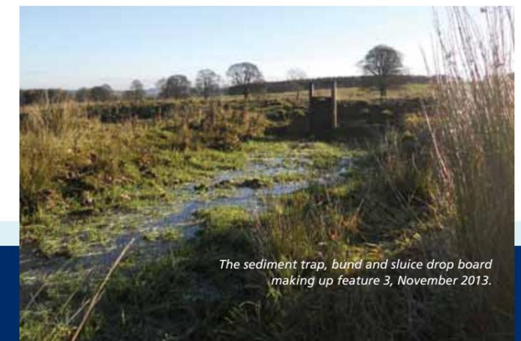
The sediment trap, bund and sluice drop board making up feature 3, November 2013.
