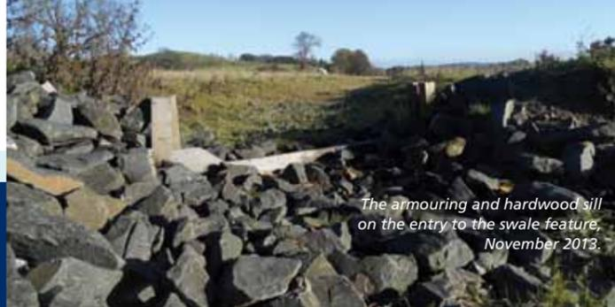
The armoured and hardwood sill on the entry to the swale feature, November 2013.
