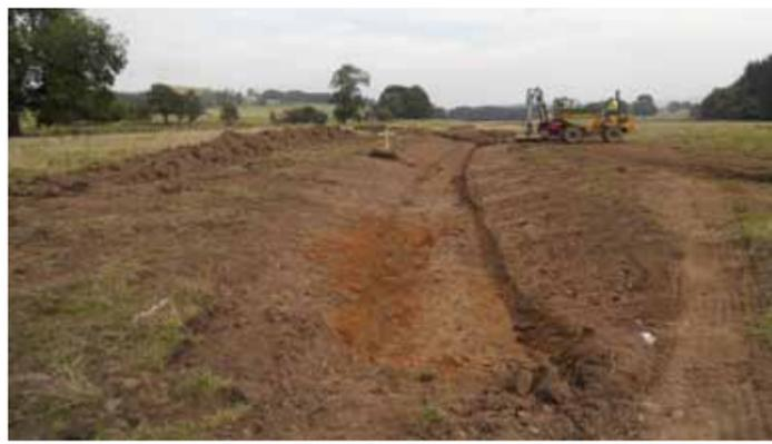
Work underway on the creation of the swale following detailed levels surveys, October 2012.
