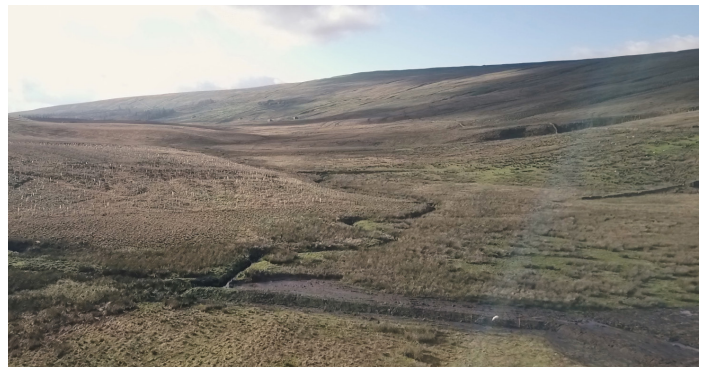
One of the Low Level Earth Bunds from the sky installed at Swarthghyll Farm on Oughtershaw Beck.
